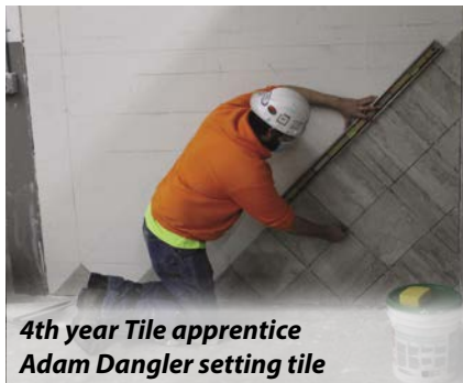
Tile Setter and Finisher apprentices working with Schluter products
