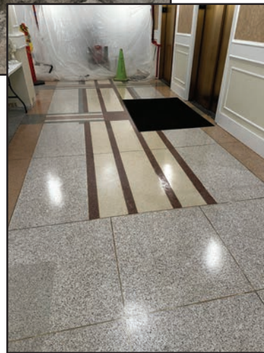
DeSpir's Keith Trode & Ryan Nichols patching Terrazzo at Brisbane Building's Lobby
