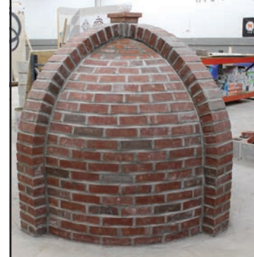
Mike Szymanski and Nathan Kent working on brick arches for a dome
