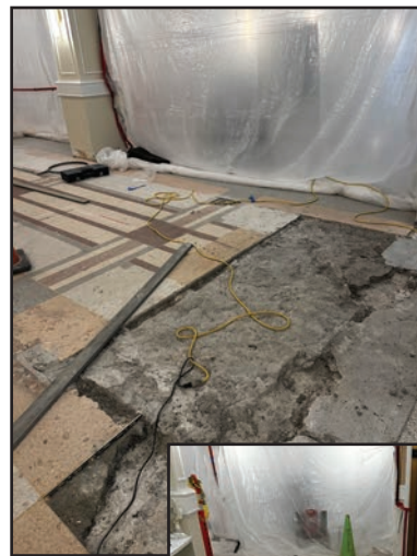
DeSpir's Keith Trode & Ryan Nichols patching Terrazzo at Brisbane Building's Lobby
