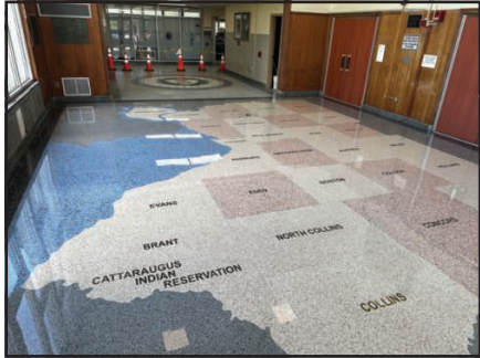
DeSpirt Mosaic's Keith Trode & Ryan Nichols Upgraded Entranceway at ECC North with Epoxy Terrazzo
