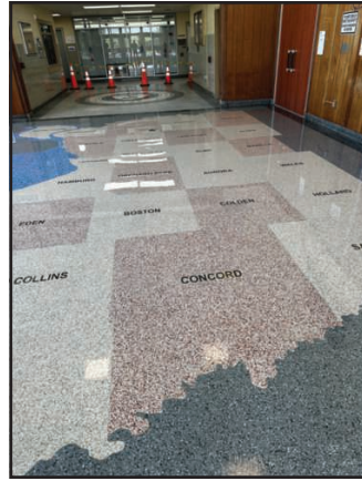
DeSpirt Mosaic's Keith Trode & Ryan Nichols Upgraded Entranceway at ECC North with Epoxy Terrazzo
